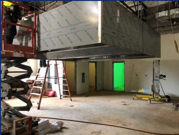
Kitchen hood system being installed
