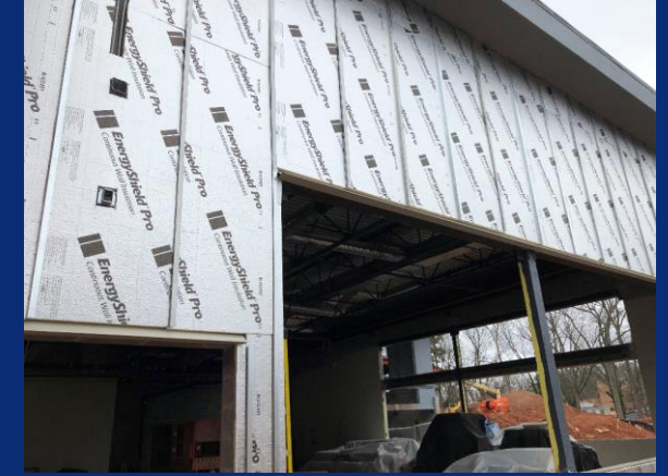
Metal panel insulation and z-furring
