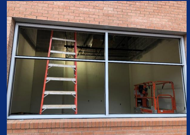
Storefront install in progress
