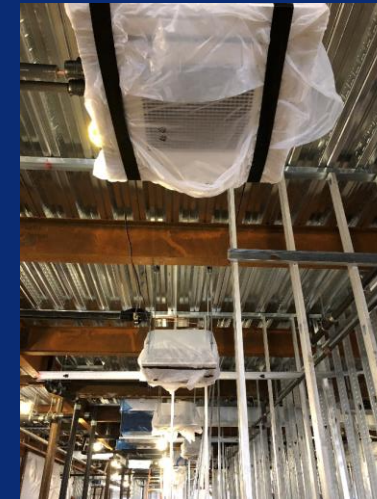
VRF units installed on main level; spiral duct being installed in lower level
