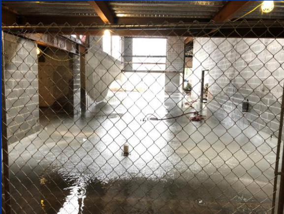
Lower level polished water cured and protected from traffic
