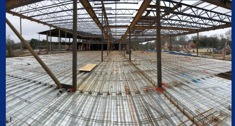
2 nd level east prepped for elevated slab pour
