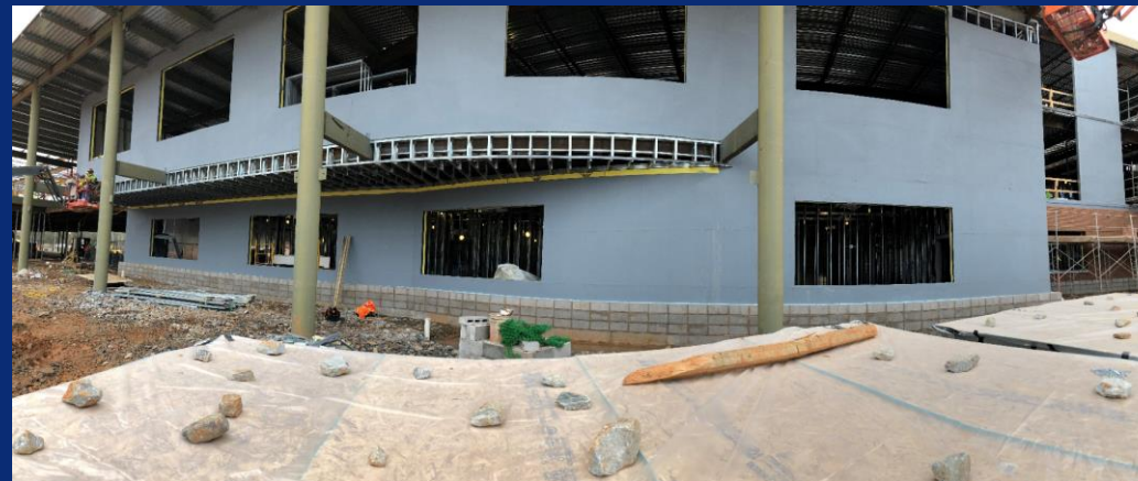
North elevation of main and 2 nd west treated with fluid applied air barrier
